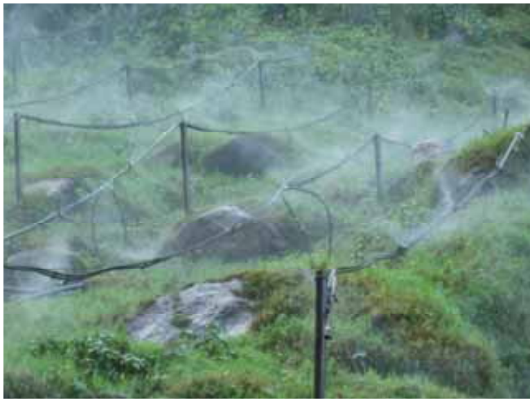
Installed artificial sprinklers at one of the three spray wetlands toad habitat at Kihansi
