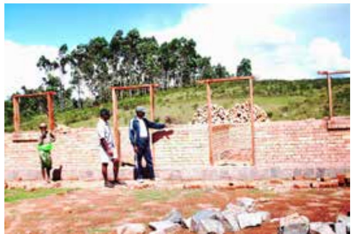
Fig. 3. School construction under progress.
